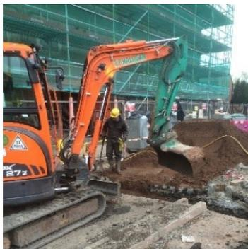
The bore field consists of 14 x 183m deep x 153mm bore holes using the highly innovative Ryan coaxial system imported from the United States. This system provides the source supply to the 100 heat pumps installed in apartments. Bore holes were positioned within the rear parking area delivering a system that limits disruption to residents. Others quoted up to 60 bore holes for the same project using fixed speed compressors.
